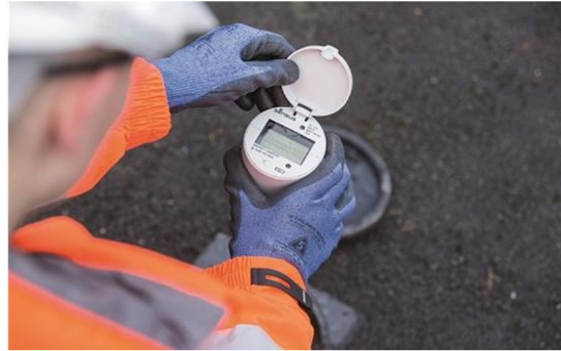
Image 4: Fitting a water meter
